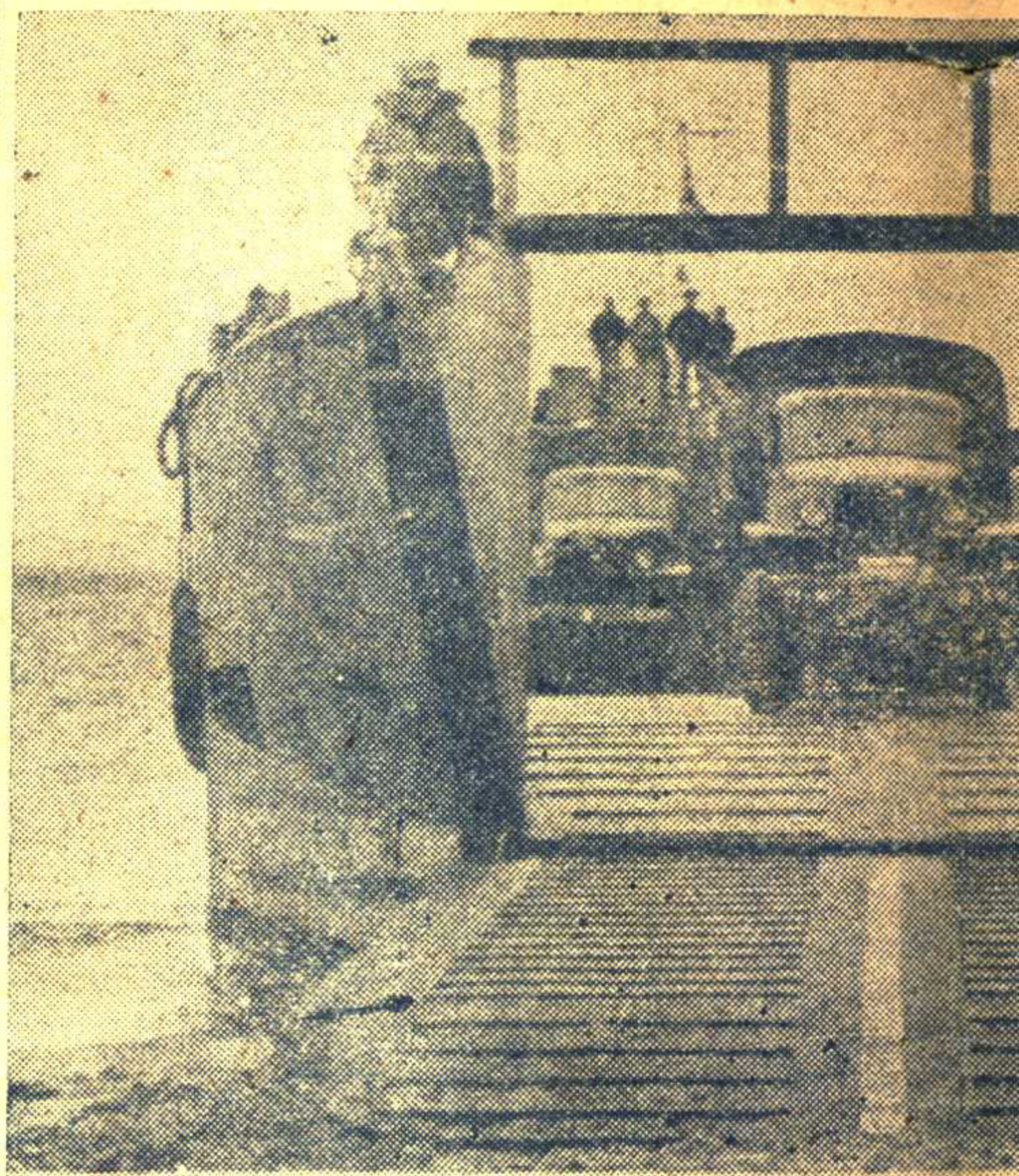
LCT is used for landing heavy tanks or the main mode of operation aboard an LST or a cargo ship.
