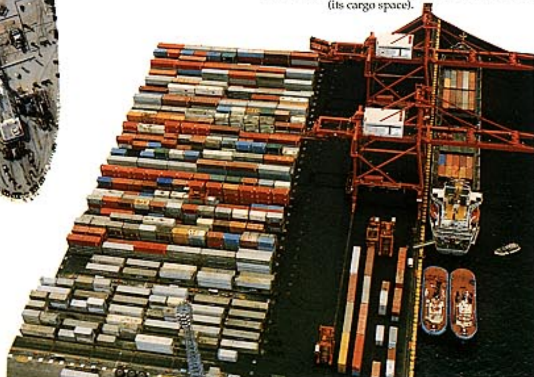
CLEVER PACKAGING This is the container port at Hong Kong. Putting goods into standard size containers has revolutionised cargo handling. Giant cranes lift the sealed containers off the ship and drop them on the shore or straight onto waiting lorries.
