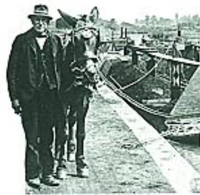
ONE HORSE POWER Towpaths were laid alongside the canals built in Britain in the 18th and into the 19th centuries, so that the narrow barges could be towed by horses.
