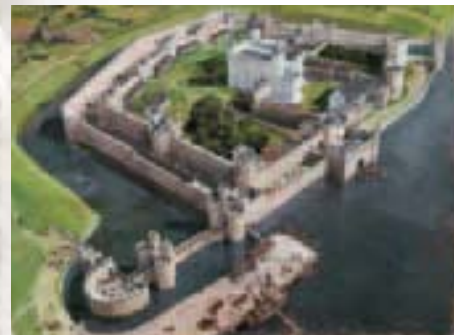
The outer curtain wall and the moat were both in place by 1300. It was now a concentric castle, because it had a double wall.
