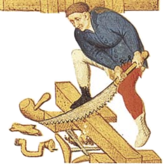
Worker cutting a beam in two with a saw
