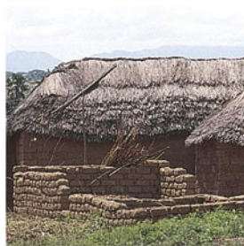
Mud bricks being used to build a house near the Jos Plateau, Nigeria
