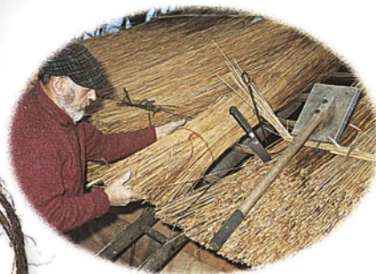
Steel sway holds reeds in place
