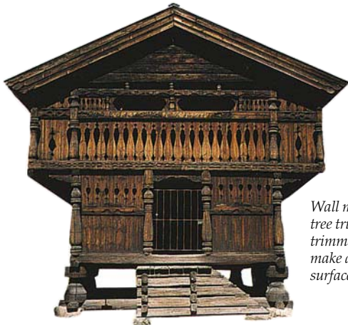
WOODEN BARN Farm buildings such as this traditional barn near Oslo, Norway, are often made of wood. This barn is raised on wooden pillars, and the sides are cut in an elegant pattern. These holes ensure good ventilation, and the pillars and overhanging roof keep out the damp and help prevent pests from eating the contents.
