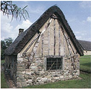
CRUCK FRAME This is the simplest wooden frame. Shaped like an inverted V, the cruck frame consists of two timbers made from the same tree trunk, so that they match exactly. These timbers are visible at both ends of this typical cruck-framed building.
