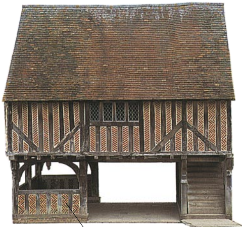
Bricks are laid in a herringbone pattern
