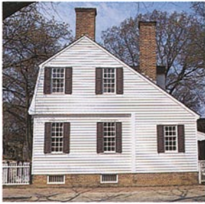
BOARDED UP Horizontal boards, called clapboard siding, or weatherboarding, cover the sides of this house in Williamsburg, Virginia. The technique gives extra protection against the elements, and makes the interior warmer.
