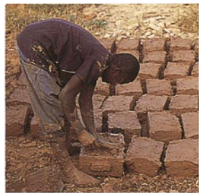
Manufacturing mud bricks in a wooden mold, Kano, Nigeria
