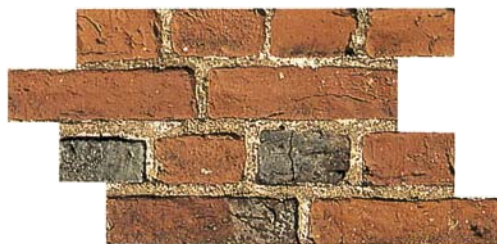
English cross bond (a header-and-stretcher bond)
