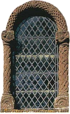
ROUNDED OPENING Window frames were not just functional but served an elaborately decorative purpose in their own right. This 12th-century round-headed window frame is carved with the heads of mythical beasts. Miniature columns, called shafts, support the arch of the window opening.
