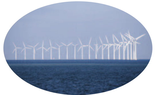
Offshore wind farm
