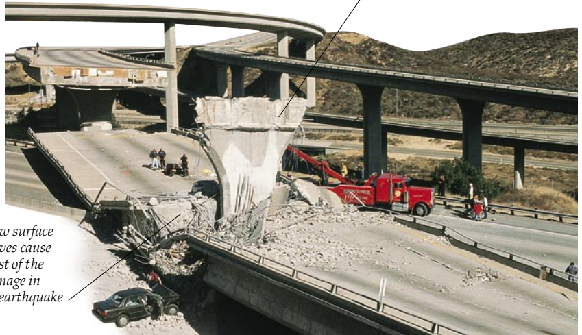
A section of road collapses as an earthquake strikes Los Angeles in 1994
