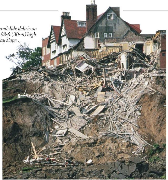
MOVING MUD When water and soil mix on a hillside, gravity pulls the mud and anything else in its path downward. Part of this hotel in the coastal resort of Scarborough, England, slipped downhill during a landslide in June 1993.
