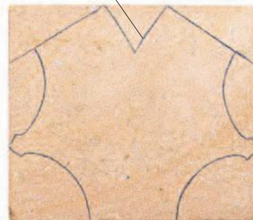
Modern masons mark out a block with pencil lines
