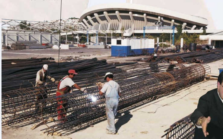
Construction work in Athens for the 2004 Games
