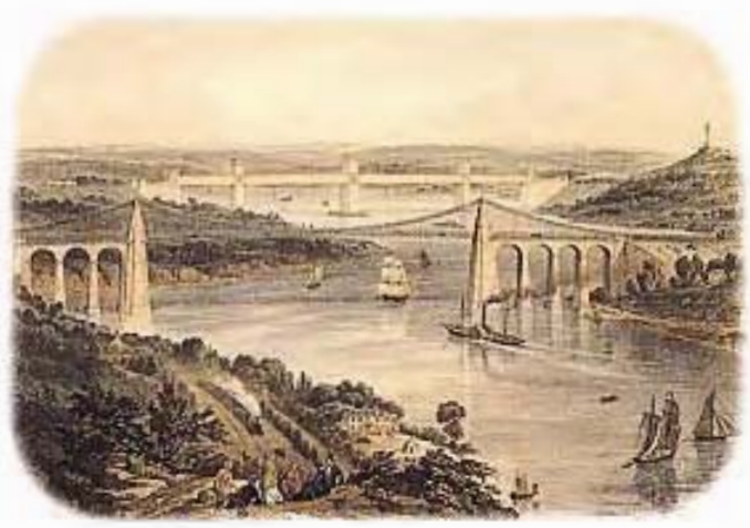
The Menai suspension bridge in Wales
