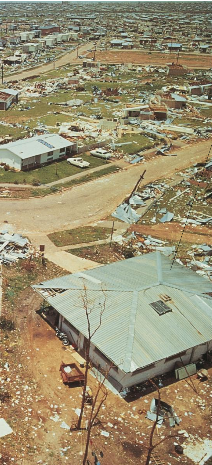
A low, flat, and well-secured roof helped this house to survive almost entirely intact
