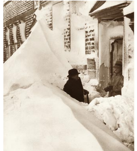
PILED HIGH Snow has piled up against the side of this house in Derbyshire, England, obscuring ground-floor windows and making it difficult to reach the front door. Snowdrifts, such as this, form when snow carried by the wind is stopped in its tracks by an obstacle.
