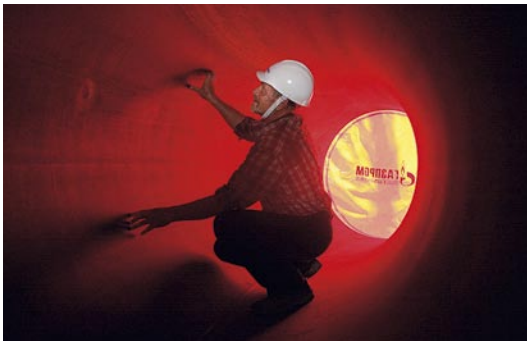
Worker inspecting a natural gas pipe, Russia
