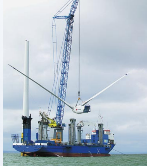
Most wind turbines resemble aircraft propellers
