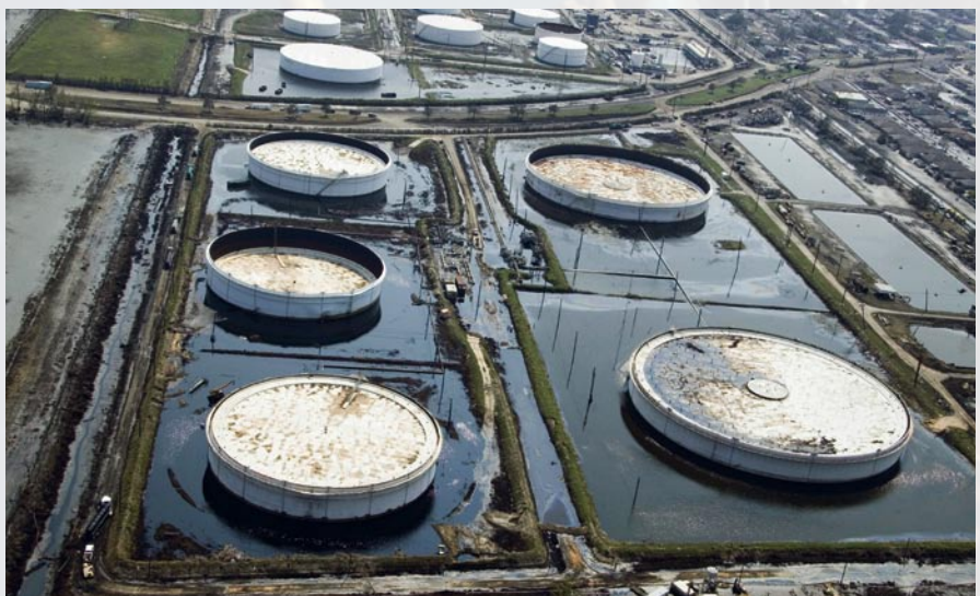
A flooded oil installation in the US hit by Hurricane Katrina in 2005
