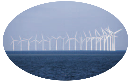
Offshore wind farm
