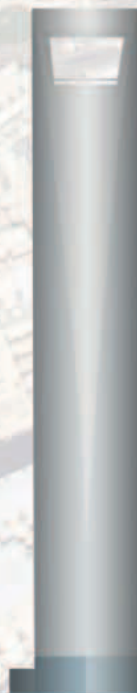
Shanghai World Financial Center, Shanghai, China Built 2008, 1,614 ft (492 m)
