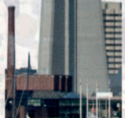
CN TOWER, TORONTO, 1973-76 This broadcasting tower was the tallest in the world until 2007, when Burj Khalifa, Dubai, surpassed it.
