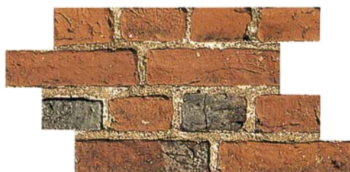
English cross bond (a header-and-stretcher bond)
