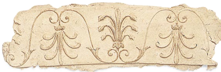
The compo molding for a fireplace
