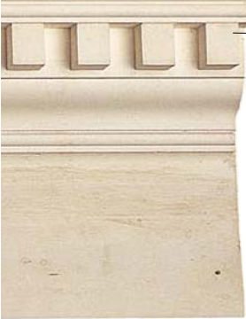
Toothlike decorations called dentils in the style of an ancient Greek cornice
