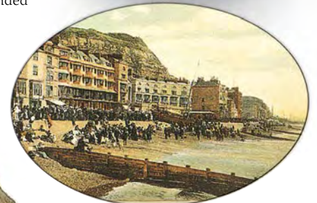
PROTECTING THE BEACH Man-made jetties keep pebbles and sand from drifting.
