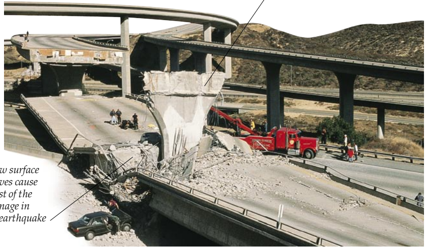
A section of road collapses as an earthquake strikes Los Angeles in 1994
