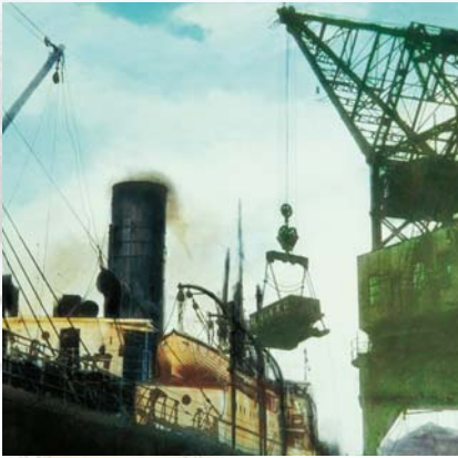
Loading coal at the docks
