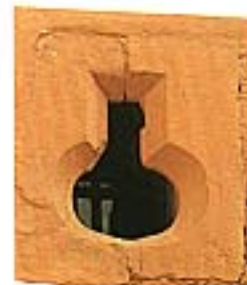
GUN PORT In the late 14th century keyhole-shaped gun-ports appeared. Round ports were usually for handguns while horizontal slots were for small cannon mounted behind walls. This example is from the Pfalzgrafenstein in Germany.
