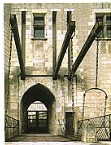
Pedestrian and main lifting bridges at Langeais, France
