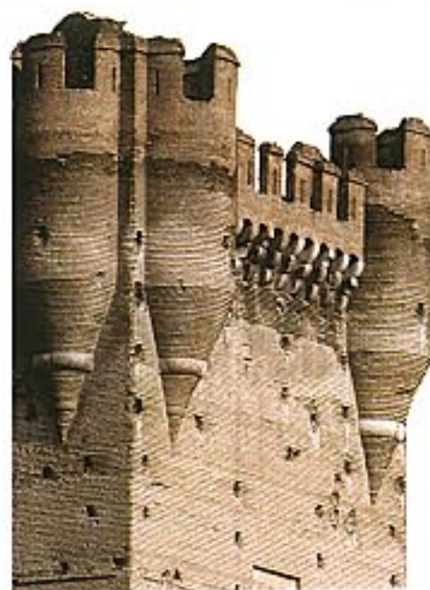
MACHICOLATIONS Machicolations were stone versions of wooden hoardings and appeared in the 12th century. The battlements jutting beyond the walls and were supported on stone corbels. Gaps left between the corbels allowed offensive material to be dropped on enemies at the wall base.
