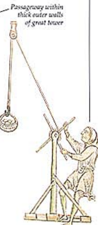
PULLEY A 13th-century mason uses a pulley to haul up a basket full of stone.
