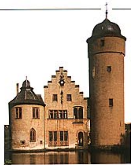
LONG OCCUPATION Schloss Mespelbrunn at Spessart, Bavaria, began as a medieval castle and was rebuilt in the 16th century to suit the taste for more comfort. Because the castle sits in a huge moat, its builders could put large windows in the outer walls.
