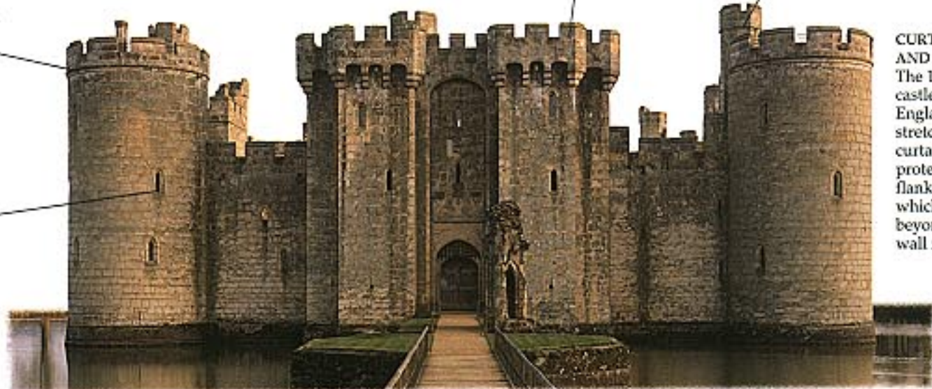
Round tower, less vulnerable to miners than sharp angles
