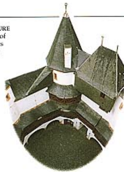
A CASTLE RE-USED The hexagonal enclosure of the Pfalzgrafenstein was added between about 1338 and 1342 to create a turret fortress, a type of castle typical of western Germany. Useful even after the end of the Middle Ages, it was strengthened further in 1607, when one end was given a protruding bastion.
