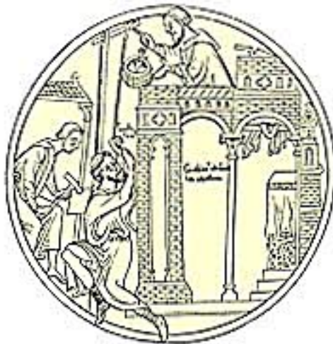
STONE ME A 13th-century mason wearing a cloth coif on his head shapes stone blocks while a basket of stone is sent up to the workman waiting at the top of the building.
