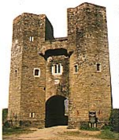
GATEHOUSE In this example the passage is flanked by huge towers. Missiles could be dropped on an attacker through slots over the arch.
