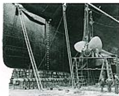
FIT FOR A QUEEN Each of the Queen Mary's (p. 55) four propellers was 5.5 m (18 ft) in diameter and weighed 35 tonnes. Cast in London, the monster screws were then shipped to a yard on the River Clyde for fitting.
