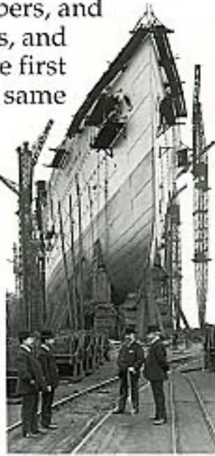
ON THE STOCKS To allow easy access and an easy launch, the hull of a ship under construction is held in place by wooden supports called stocks. This picture shows the luxurious liner the Aquitania (pp. 54–57) in 1913. She was launched, stern first, into the River Clyde in Scotland a few weeks later.
