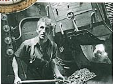
STOKING THE FIRE A fireman on a small steamer stokes the furnace to create the steam. A big liner had more than 180 firemen, each feeding 5 tonnes of coal into the furnaces every day.
