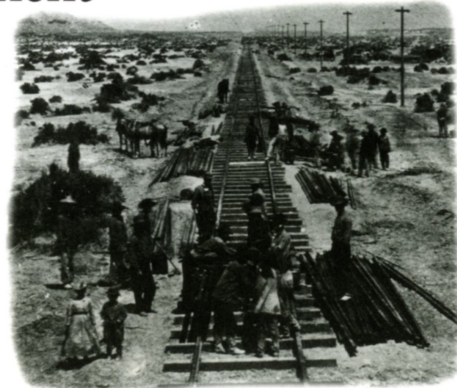
STRAIGHT TO THE HORIZON With visitors looking on, a Chinese work gang for the Central Pacific Railway lays track across the desert in the mid-1860s. The earth for the roadbed was shaped, then wooden cross-ties laid, and iron rails were placed on top. Spikes were hammered into the wood to clamp the rails in place.
