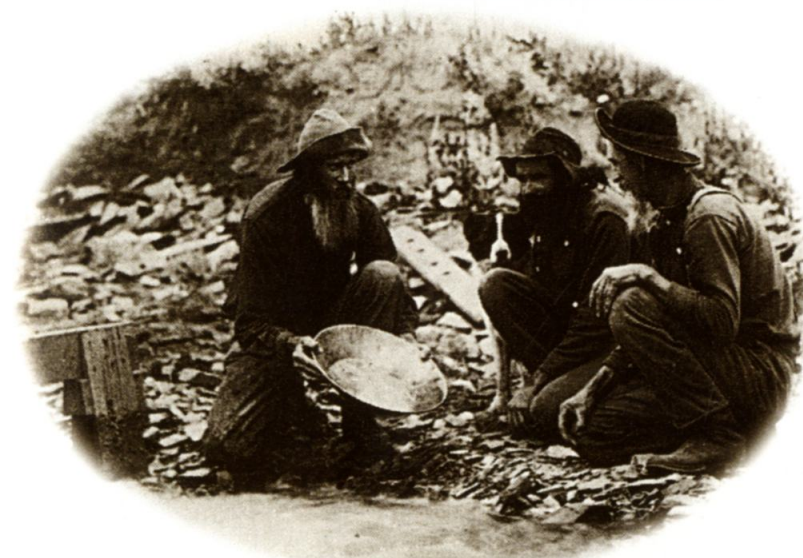
CHILLY, WET, AND SLOW About 1878, Dakota Territory miners slosh silt around in their shallow pans until the heavier gold dust is left. Washing gold required robust health and much patience, for the stream water was ice cold and the process tedious.
