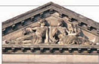
Allard Pierson Museum's Neo-Classical façade made of Bremer and Bentheimer stone
