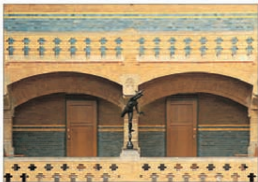
Decorative brickwork on the façade of the Beurs van Berlage
