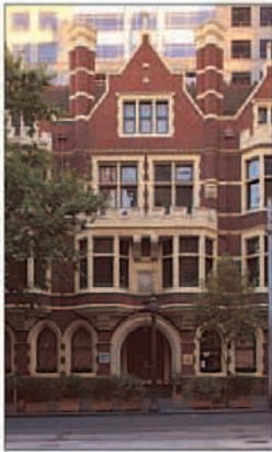
Chambers at No. 120 Collins Street
