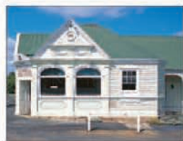
Typical 19th-century building in Bothwell
