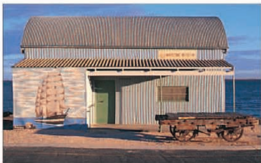
Former timber shed now home to the Maritime Museum, Port Victoria
