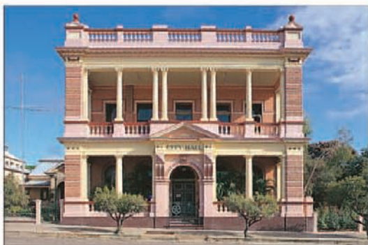
Ornate 19th-century façade of City Hall in Charters Towers
