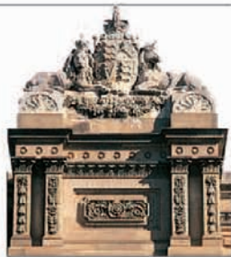
Detail of the ornate front parapet of Edmund Wright House
