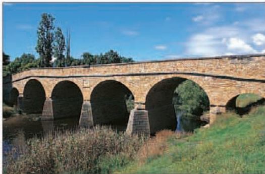
Richmond Bridge, constructed with local sandstone
