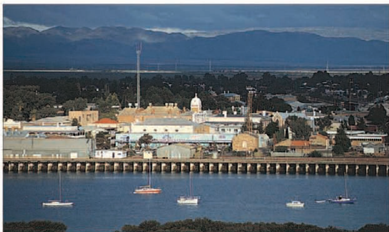
Harbour view of Port Augusta, backed by its power stations
