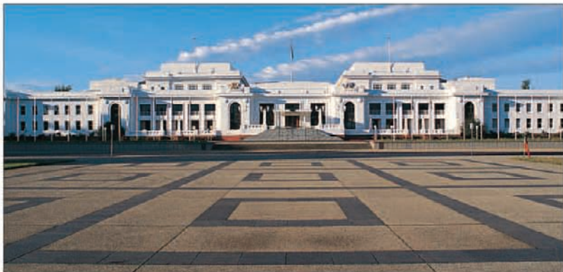
Neo-Classical façade of Old Parliament House and its impressive forecourt
