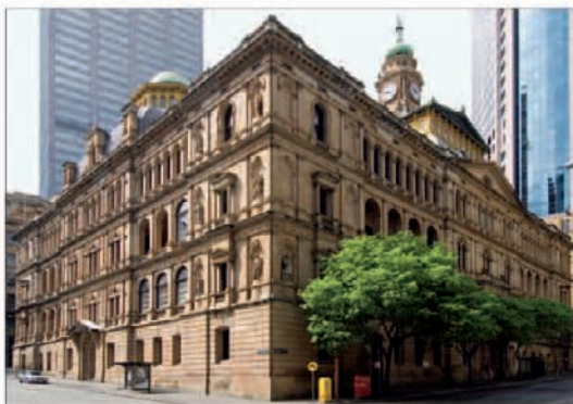
The imposing sandstone edifice of the Lands Department Building
