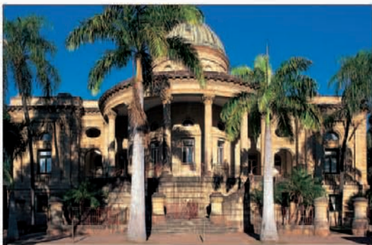
Facade of Customs House on Quay Street, Rockhampton
