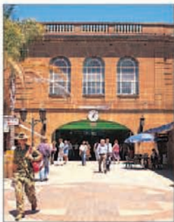
Pedestrian concourse outside Central Railway Station
