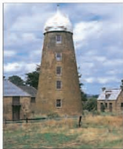
Distinctive façade of the Oatlands Flour Mill
