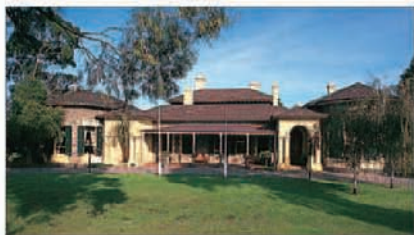
Front of the house viewed from North Terrace
