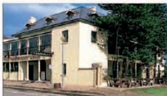
Windsor is one of the best preserved 19th-century towns in the state. The Macquarie Arms Hotel is considered to be the oldest operational hotel in Australia (see p168).
