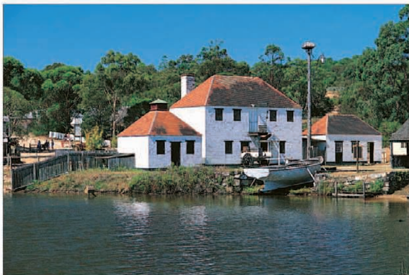
Preserved 18th-century Custom House at Old Sydney Town near Gosford
