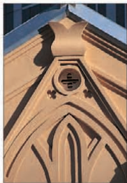
Roof detail of St Francis' Church
