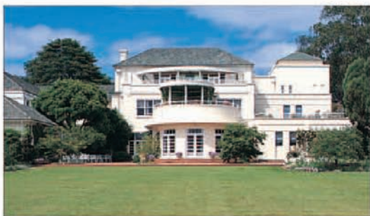
Elegant façade and front grounds of Government House
