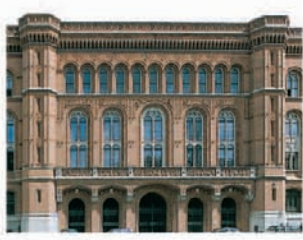
Southern façade of the Berliner Rathaus
