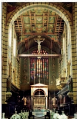
The 1920s interior of Mosteiro São Bento, with its painted ceiling
