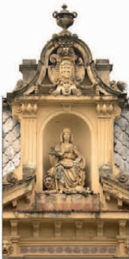
Detail on the façade of Palácio Rio Negro
