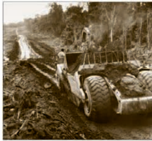
Trans-Amazon Highway construction near Altamira Brazil, July 1971
