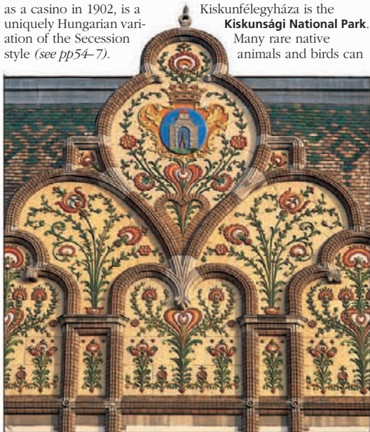
Detail of the ornate Town Hall façade at Kiskunfélegyháza
