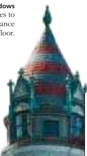
Queen Anne turret topped by a finial at No. 1015 Steiner Street
