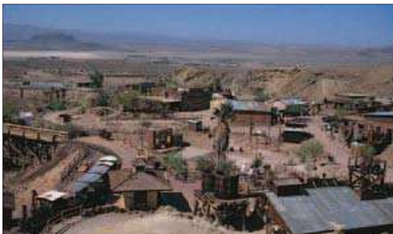
Restored and reconstructed buildings in Calico Ghost Town
