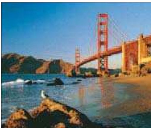
Golden Gate Bridge, San Francisco
