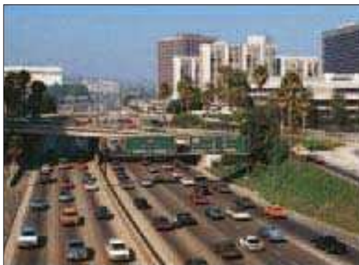
Traffic on the Harbor Freeway, Los Angeles
