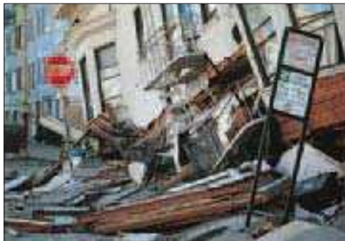
Destruction caused by the Loma Prieta earthquake
