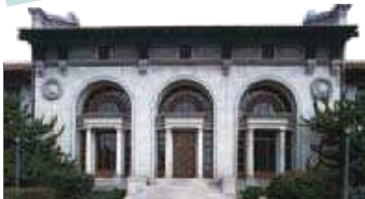
The Hearst Mining Building around the Mining Circle ⑨
