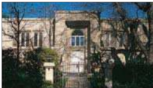
Faye Dunaway's house at No. 714 Palm Drive ①
