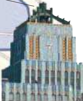
Eastern Columbia Building (1930) This Art Deco building, designed by Claude Beelman, is one of the most impressive of its kind in LA.
