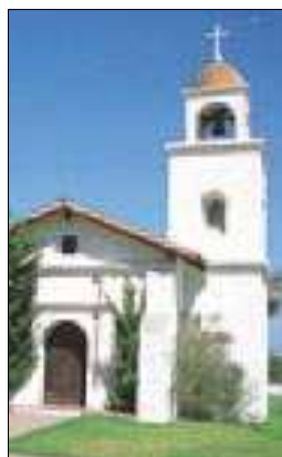
Reconstructed façade of Santa Cruz Mission
