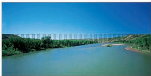
High Level Bridge over the Oldman River, Lethbridge
