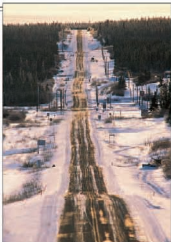
The Alaska Highway in winter is often covered in snow and affected by frost heave. Since it was opened to the public in 1949, teams of maintenance workers have ensured that the road is open year round.
