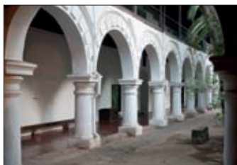
Colonnaded passageway bordering the yard at Convento de San Francisco (see p68), Santiago
