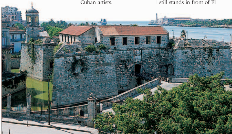
View of the Castillo de la Real Fuerza: the drawbridge and entrance, the moat, and the Giraldilla tower (left)
