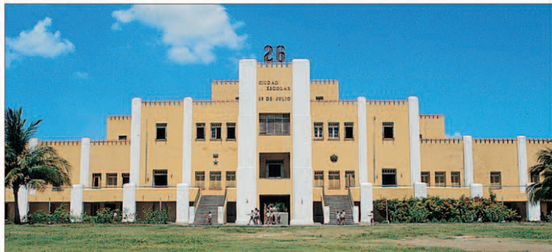
The impressive façade of the former Moncada army barracks, now a school and museum
