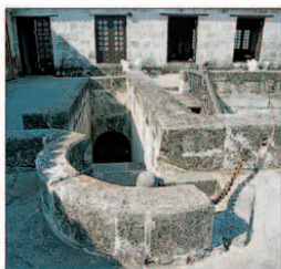
Stairway leading to the battlements, Castillo de la Real Fuerza
