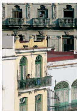
Restored buildings around Plaza Vieja, Havana
