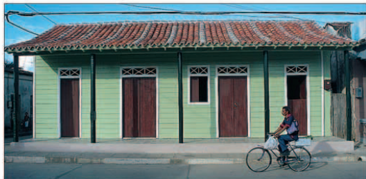
A typical single-storey wooden house in Baracoa
