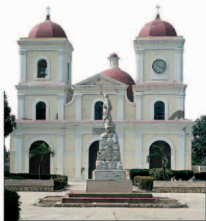
Facade of the Iglesia de San Fulgencio at Gibara
