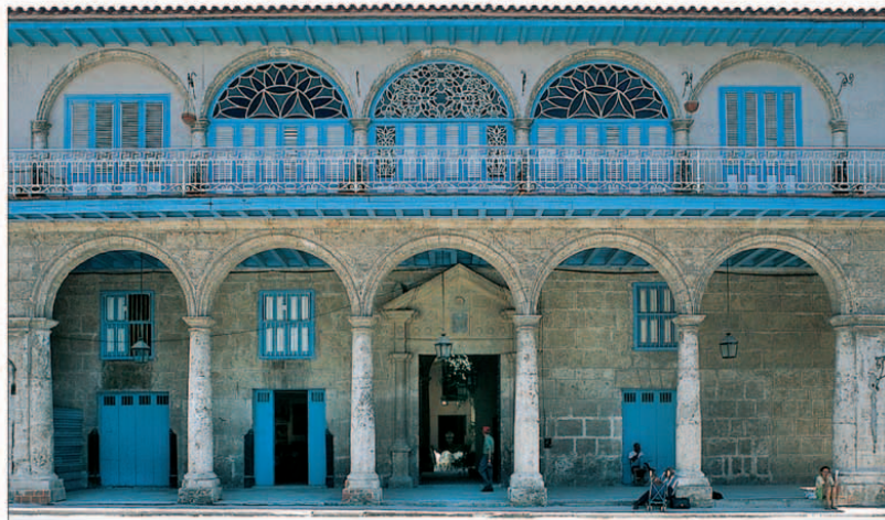
Façade of Casa del Conde Jaruco, with typical mediopunto stained-glass windows on the first floor
