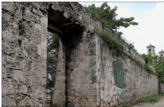
Remaining section of the old City Wall near Estración Central
