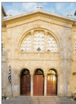
The façade of Agios Kendas church, which was built around 1930
