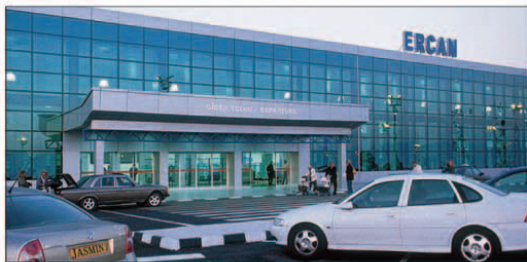
Airport terminal building at Ercan, North Cyprus
