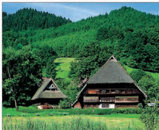
The Vogtsbauernhof in Gutach, the oldest house in the Black Forest
