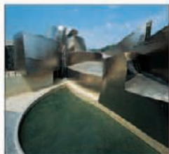
1997 Astonishing sculptural forms used by American architect Frank Gehry for new Guggenheim Museum in Bilbao (see p304)
