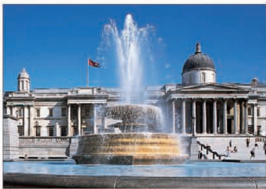
The Trafalgar Square façade of the National Gallery
