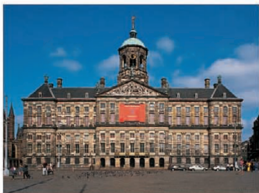
The splendid Classical façade of the 17th-century Koninklijk Paleis
