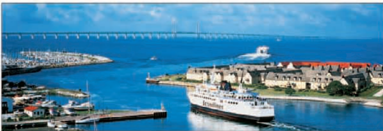
The newly constructed Öresund Link, spanning the Öresund channel
