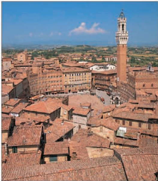
Aerial view of Siena's Piazza del Campo and surrounding palazzi
