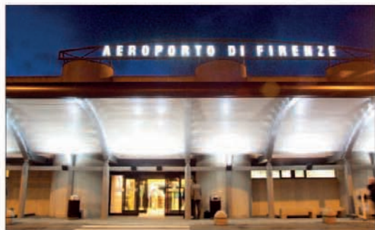
Modern exterior of Florence's Amerigo Vespucci airport
