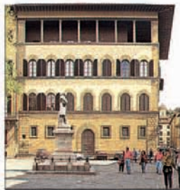
The façade of Palazzo Guadagni
