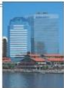
High-rise architecture in downtown Jacksonville
