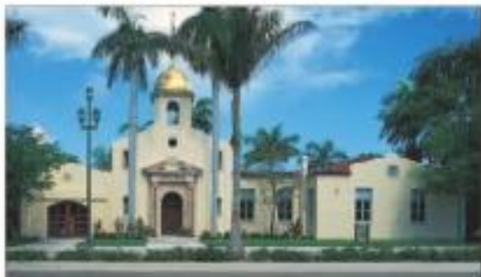
Boca's attractive town hall, designed by Addison Mizner and built in 1927
