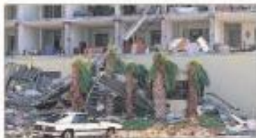
An apartment building after its façade was ripped off by Andrew's ferocious winds
