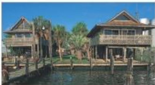
Restored houses on the water's edge in Water Street, Apalachicola
