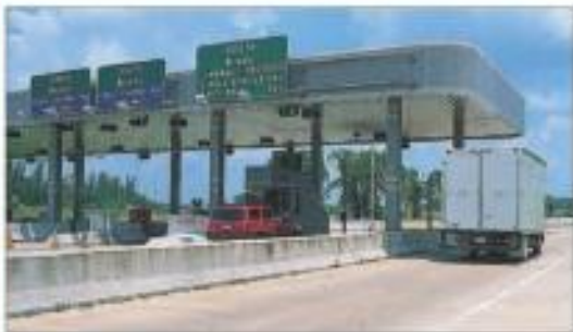
The toll plaza on Florida's Turnpike at Boca Raton
