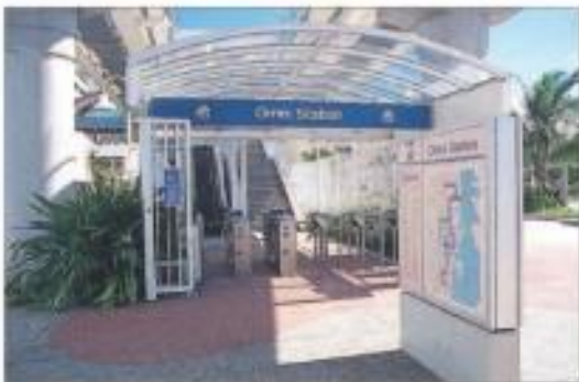
A typical Metromover station, with a plan of the network by the entrance
