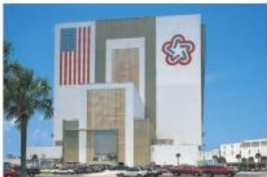
The Vehicle Assembly Building, which dominates the flat landscape
