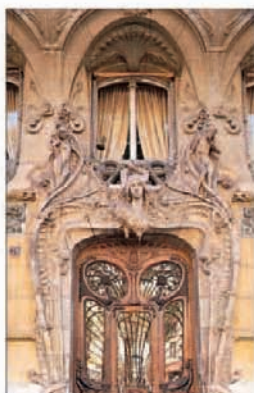
Original Art Nouveau doorway at No. 29 avenue Rapp
