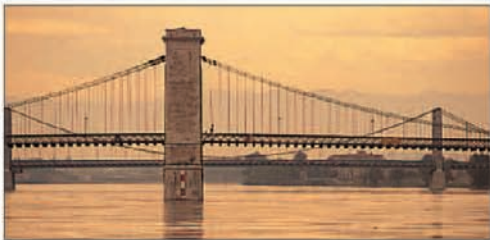
Suspension bridge over the Rhône at Tournon-sur-Rhône
