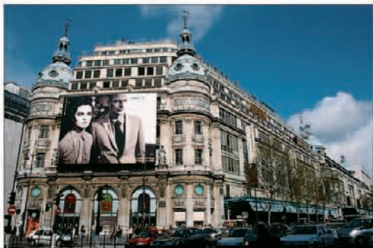
The 1865 façade of Au Printemps department store
