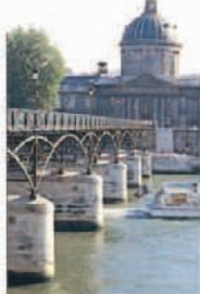
Passerelle des Arts This steel reconstruction of Paris's first cast-iron bridge (1804) was inaugurated in 1984.
