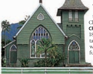
The striking facade of Wai'oli Hui'ia Church
