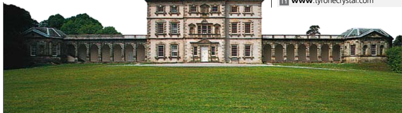
Florence Court, the former seat of the Earls of Enniskillen
