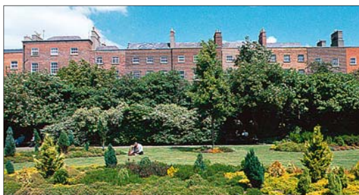
Georgian town houses overlooking Merrion Square gardens
