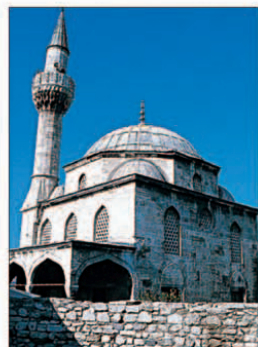
Şemsi Paşa Mosque, built by Sinan for Grand Vizier Şemsi Ahmet Paşa
