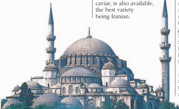
The New Mosque, a prominent feature on the Eminönü waterfront
