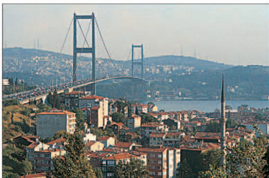
The Bosphorus suspension bridge between Ortaköy and Beylerbeyi
