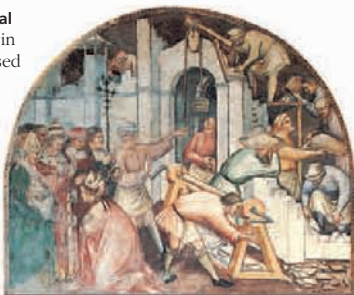
Construction of Alessandria Almost all towns were ringed with strong walls. This fresco (1407) by Spinello Aretino is a valuable record of medieval building techniques.
