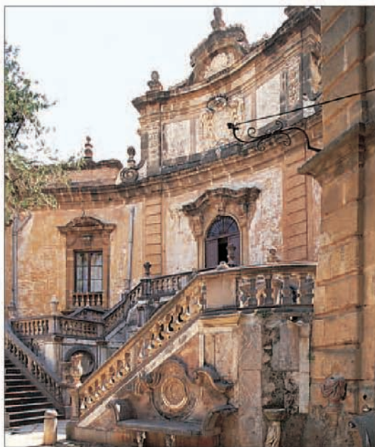
Open-air staircase of the eccentric Villa Palagonia in Bagheria
