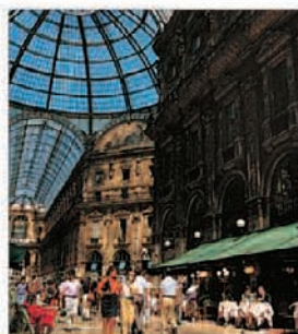
Industrial innovations in glass and metal were applied in new buildings, like Mengoni's imposing Galleria Vittorio Emanuele II (1865) in Milan (see p194).
