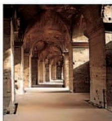
Internal Corridors These allowed the large and often unruly crowd to move freely and be seated quickly.
