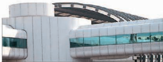
Part of the extension to Fiumicino airport, Rome
