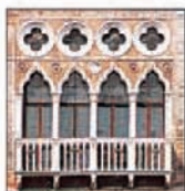
Typical Venetian Gothic window
