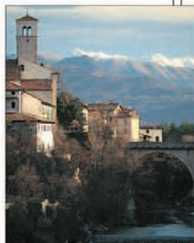
The bridge at Cividale del Friuli
