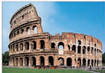
Doric, Ionic, and Corinthian Tiers The tiers inspired many Renaissance architects, who also plundered the building, using its travertine to build palaces and part of St. Peter's.
