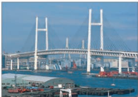
Yokohama Bay Bridge
