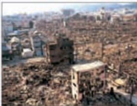
The center of Kobe in ruins following the January 1995 earthquake
