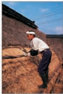
A thatcher at work replacing worn thatch
