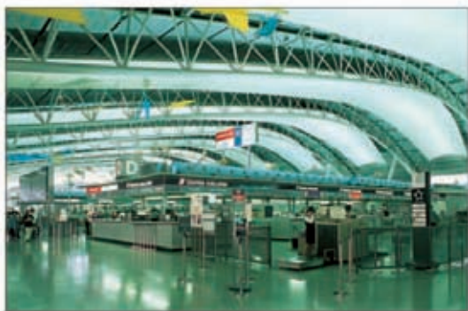
Interior of check-in lobby at Kansai International Airport
