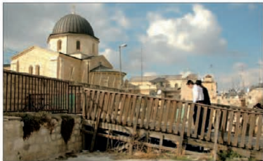
Orthodox Jews cross the rooftops of the Old City
