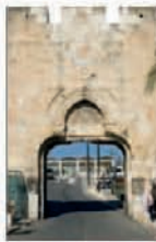
Dung Gate, leading to the Western Wall
