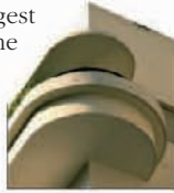
Rounded balconies on a Bauhaus building
