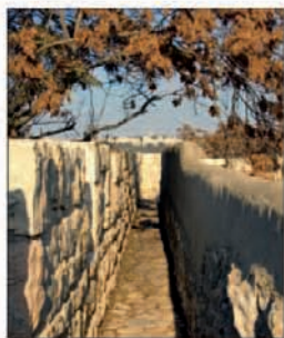
A section of the ramparts just east of New Gate ②
