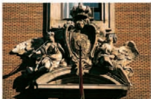
Façade detail, Real Casa de la Aduana
