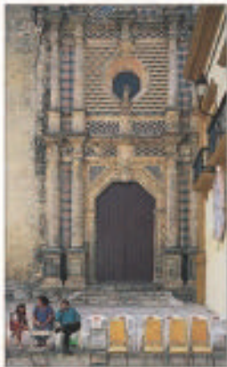
Tiled doorway of the Ex-Templo de San José, now a cultural center
