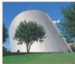
Monterrey's massive cultural complex, the Planetario Alfa
