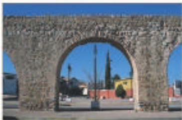
A beautifully preserved section of Chihuahua's aqueduct, which dates from colonial times
