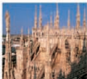
View of the roof
