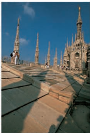
Detail of the Duomo's rooftop
