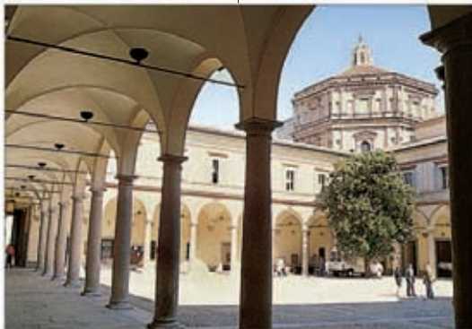
The Giuseppe Verdi Conservatory, housed in a former monastery
