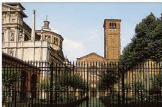
The Sanctuary of Santa Maria dei Miracoli and San Celso
