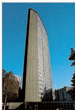
The Pirelli Building is the tallest in Milan (see p118)
