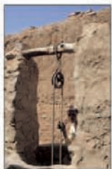
Well in the Oulad-Abdelhalim Ksar
