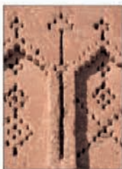
Detail of the walls of Tinerhir Kasbah
