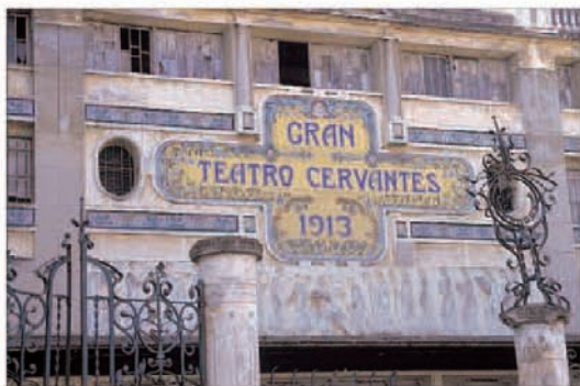
The dilapidated Art Deco façade of the Gran Teatro Cervantes
