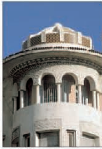
1930s building, Casablanca, dating from the Protectorate
