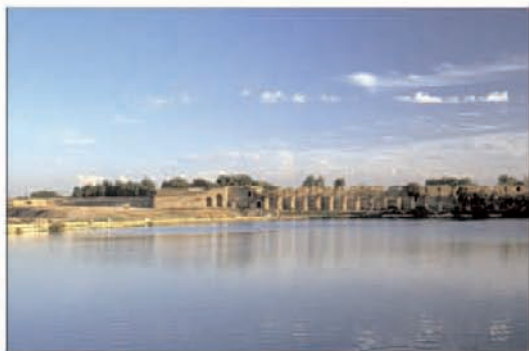
The Bassin de l'Aguedal, a water tank created by Moulay Ismail
