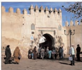
Fortified gateway into the mellah in Sefrou
