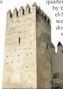
A tower set in the walls of the méchouar
