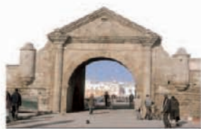
The Porte de la Marine, built by Sidi Mohammed ben Abdallah
