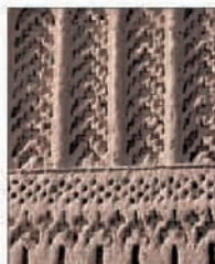
Detail of the ksar of Oulad Abdelhalim in Rissani
