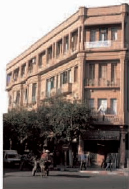
An apartment block in Guéliz, Marrakech's Ville Nouvelle
