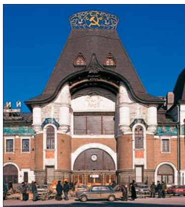
Main entrance of the Style-Moderne Yaroslavskiy station on Komsomolskaya ploshchad
