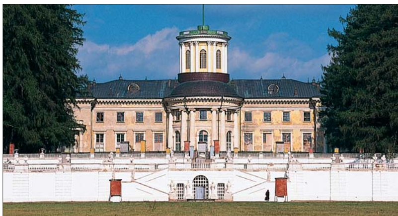
The southern, garden façade of the Neo-Classical, stucco-covered, wooden palace at Arkhangelskoe
