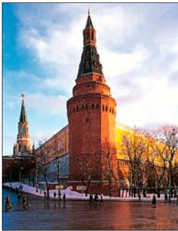
Corner Arsenal Tower with the Arsenal and Nicholas' Tower
