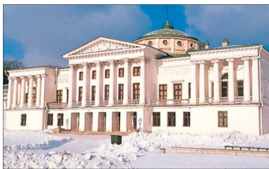
Main façade of the imposing, Neo-Classical Ostankino Palace
