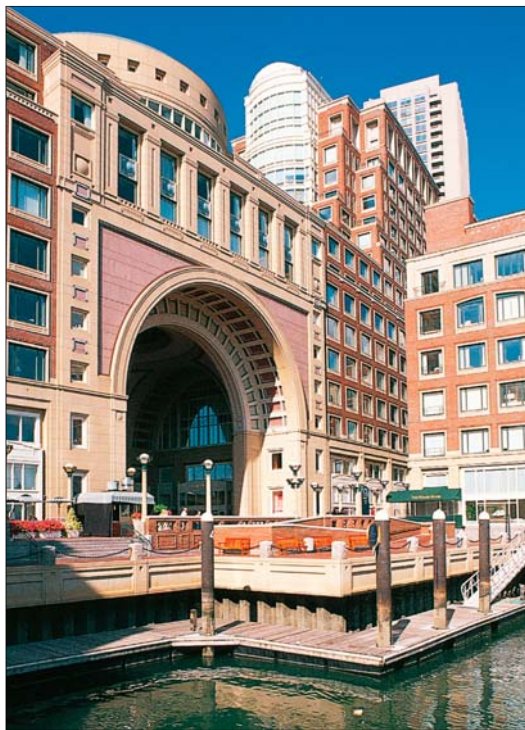
Rows Wharf development, typical of Boston's waterfront regeneration
