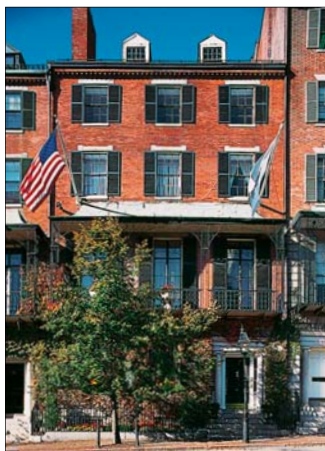
Elegant Federal-style houses on Beacon Street, overlooking Boston Common
