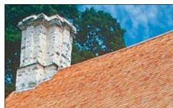
Eleazer Arnold House chimney, Providence, Rhode Island
