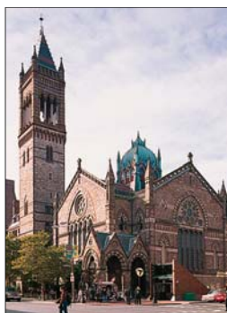
The New Old South Church on the corner of Copley Square
