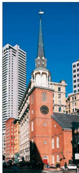
Old South Meeting House, in stark contrast to the modern city
