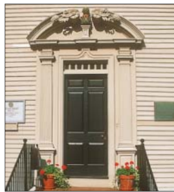
Architectural detail is typical of the Washington Square district.
