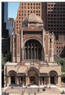
St. Bartholomew's Church
