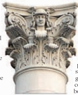
Top of a column at the US Custom House
