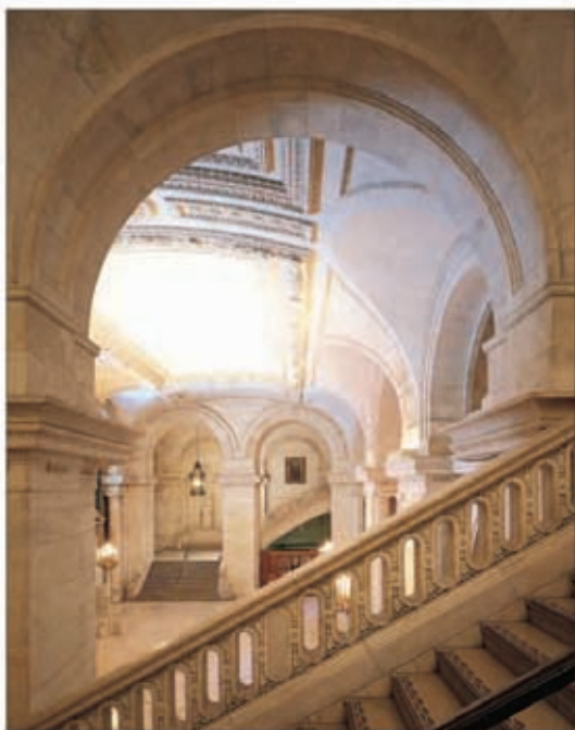
Barrel vaults of carved white marble over the stairs in the Astor Hall
