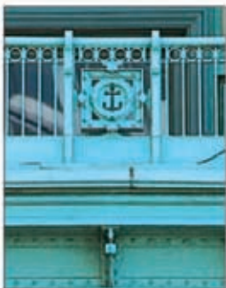
Ironwork railing on the Battery Maritime Building
