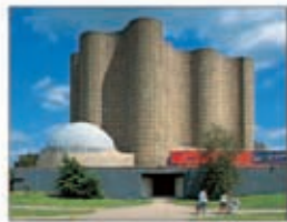
The concrete curtain wall of the New York Hall of Science
