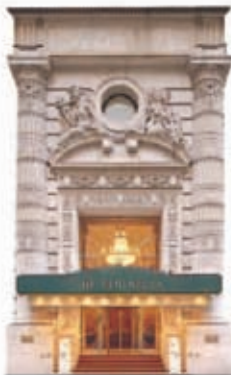
Entrance to the Peninsula Hotel (see p289)
