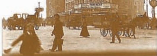
Flatiron Building during its construction
