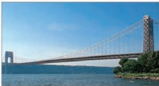
The 3,500-ft (1,065-m) span of the George Washington Bridge
