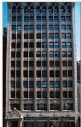
The Bayard-Condict Building
