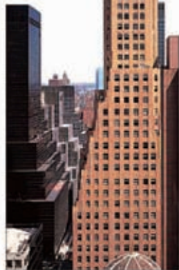
The General Electric Building on Lexington Avenue
