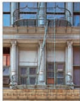
Cast-iron facade, Greene Street ⑮
