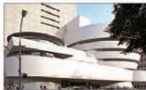
Fifth Avenue facade
