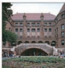
The facade on 77th Street
