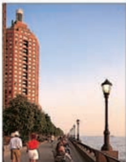
Battery Park City esplanade
