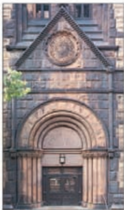
St. Martin's Episcopal Church on Lenox Avenue
