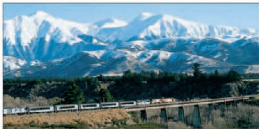
The TranzAlpine crossing Kowai Bridge near Springfield
