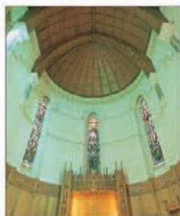
Timber ceiling in Christchurch Cathedral
