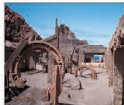
Old sulphur mining equipment on White Island
