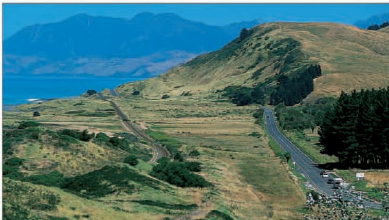
State Highway 1 paralleling the railway line along the Kaikoura coast
