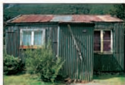
An original tunneller's cottage at Arthur's Pass village
