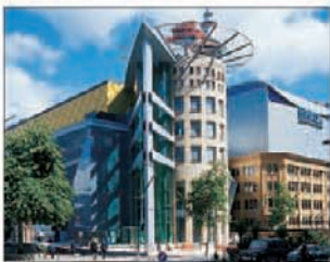
Façade of the Village SKYCITY Cinemas
