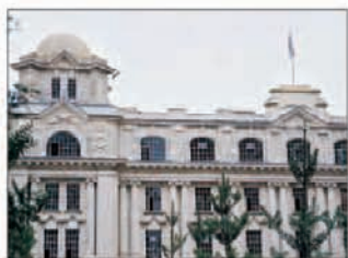
Britomart Transport Centre Auckland's public transport hub is housed in the refurbished Chief Post Office building.
