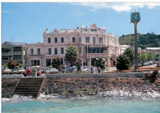
Well-preserved Victorian buildings on Devonport's waterfront
